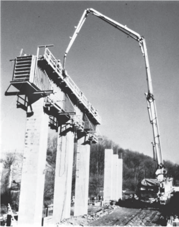
Autopista Pennsylvania Southern, Filadelfia, Pensilvania. (Cortesía de Economy Forms Corporation.)
