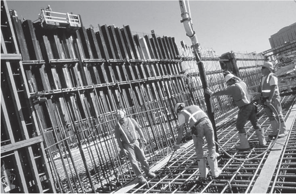
Colado del concreto, Big Dig, Boston, MA. (Steve Dunwell/The Image Bank.)
