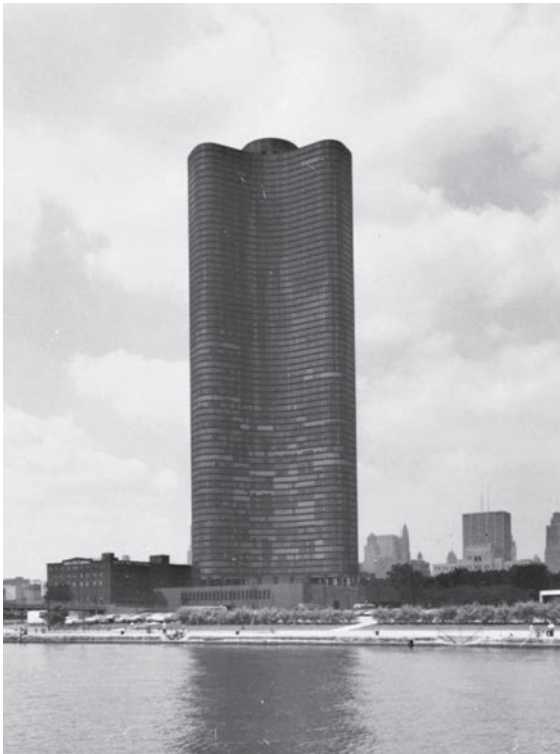
Torre Lake Point, Chicago, Illinois. (Cortesía de Portland Cement Association.)
